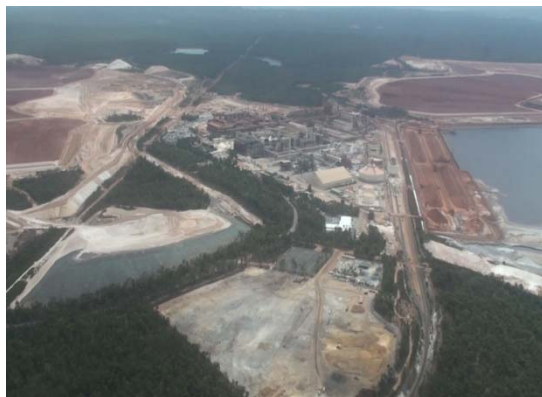
BHP – Worsley Refinery
