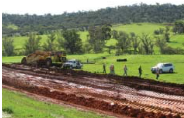
Mine haul road construction above and below
