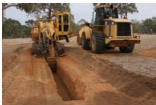
Trench digging for bulk samples left & sample collection right
