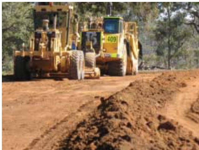
Mine haul road construction above and below
