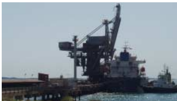
Kwinana Port bulk loading terminal above
