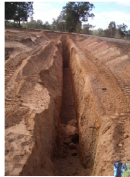
Trenching program at Bindoon North to collect bulk samples.
