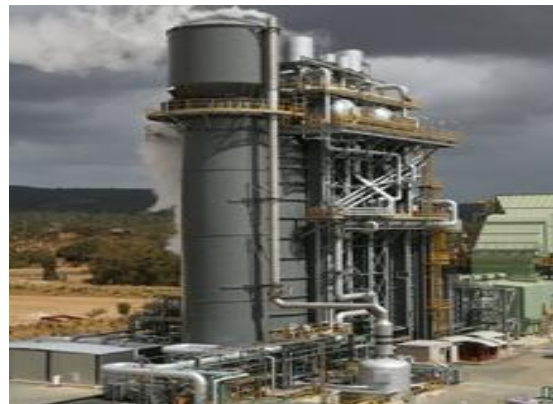
Alcoa - Pinjarra Refinery
