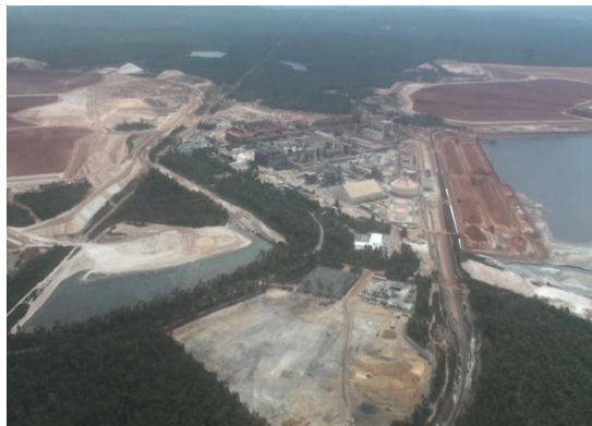
BHP - Worsley Refinery
