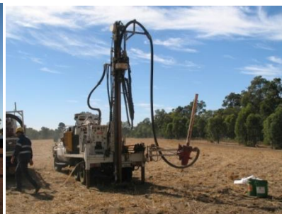
BRL Contractor Vacuum Drilling
