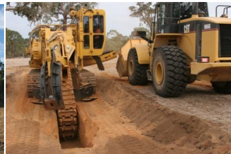
BRL's Sample Trench Drilling
