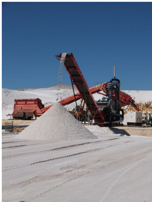
Operating Plant at Urban's Maralla Road Deposit
